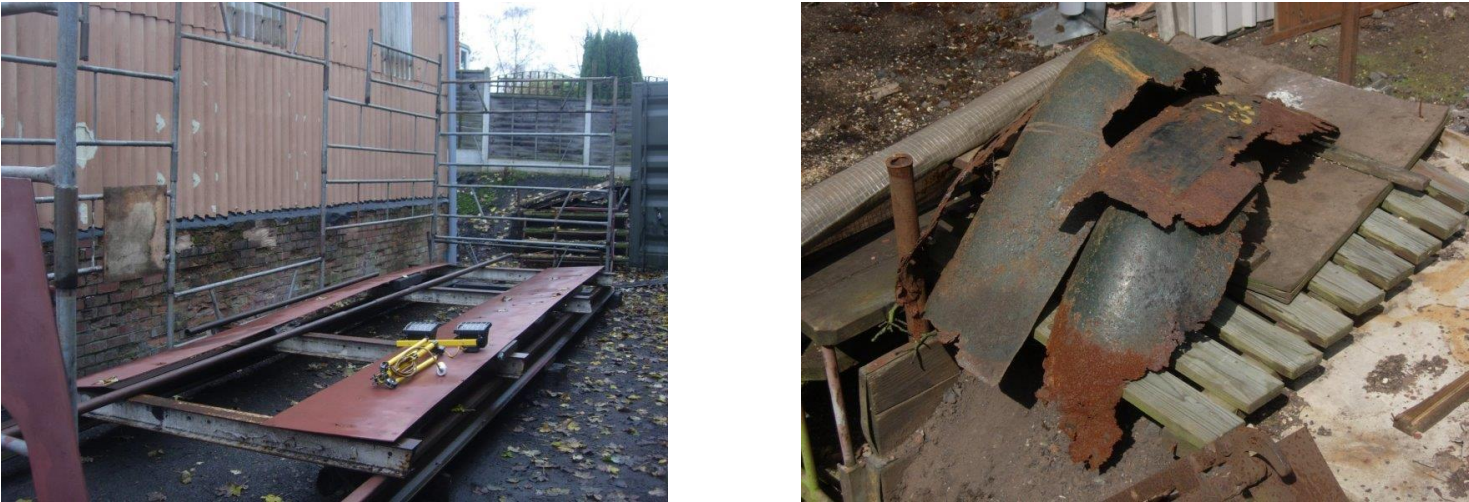
The base being laid for the first of two new side tanks and salvaged parts to be used as patterns
