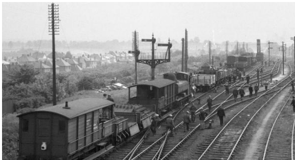
Repairs and clearance underway
