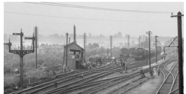
General view of damage, Down freight approaching
