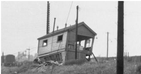
Rear view of damaged box
