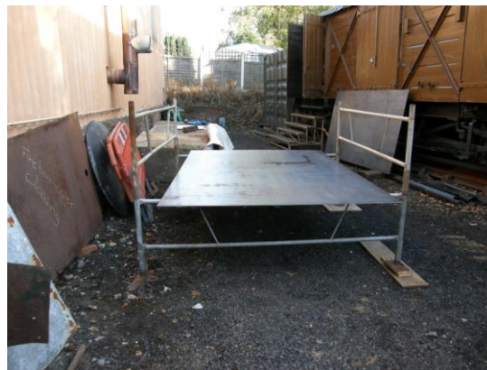
THE NEW BUNKER FLOOR JUST DELIVERED
