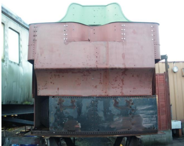
Upper section of the rear of the bunker, positioned temporarily on the old bunker. Note that the bottom halves of the old corner sheets have been carefully cut out.
